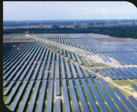
Dholera 5000 MW TATA Solar Plant
