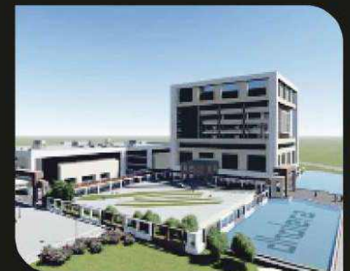
Dholera ABCD Building Single Window Clearance
