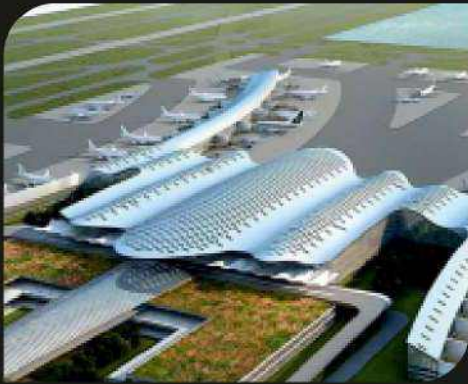
Dholera Asia's Second Largest International Airport
